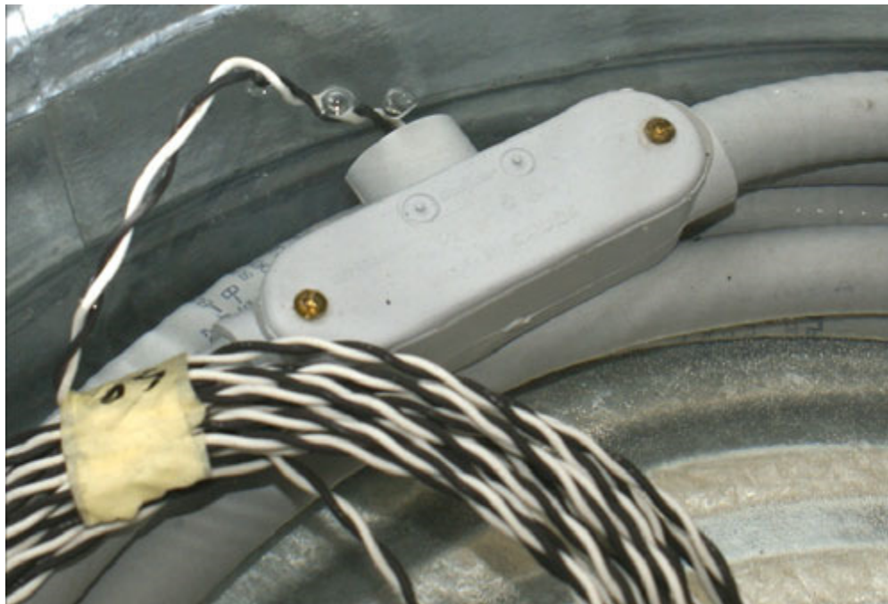
Preformed Loop with an Air Pocket
