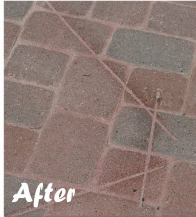
Pavers with Black Sealant and Colored Sand
