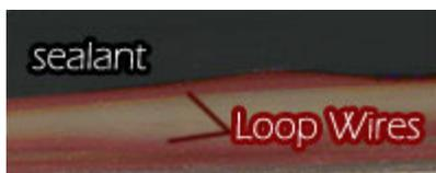
Air Pockets like the one pictured above can cause false detections or loop failure.
