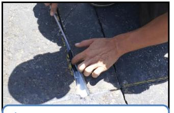
2) Gently press the yoke into the bead of sealant, the yoke should be resting on a small layer of sealant.
