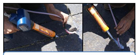
**1)** Lift the yoke up and place a bead of sealant down in the groove in the yoke area below the yoke.
