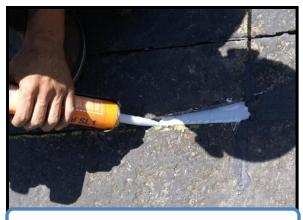
3) Seal over the yoke to fill the groove.
